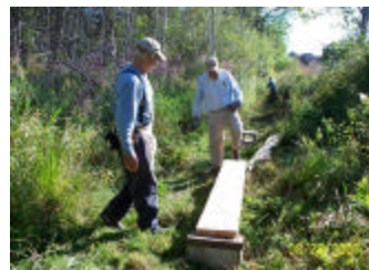
Bog Bridges being built by Trust members Steve Smith and Paul Cully at Swedes Crossing
